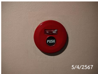
Fire Alarm Manual Station
